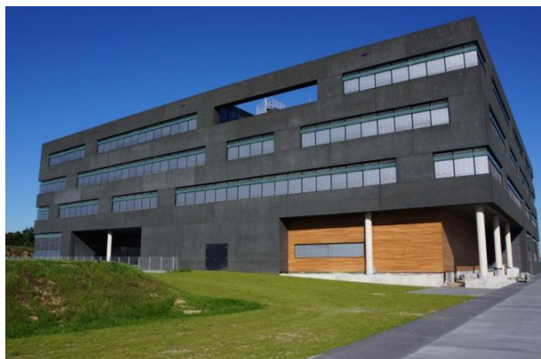
The modern CITEC building at Bielefeld University: home to an interdisciplinary collaboration between engineering and life scientists
